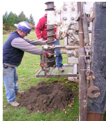
(b) drilling activities
